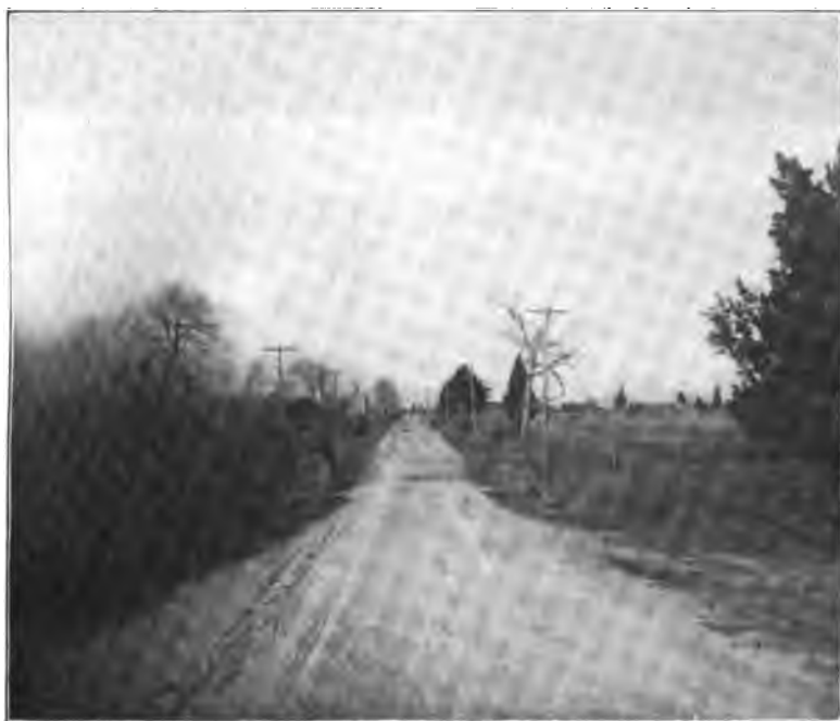
Little Egg Harbor Township County road, Ocean Co., before improvement.
